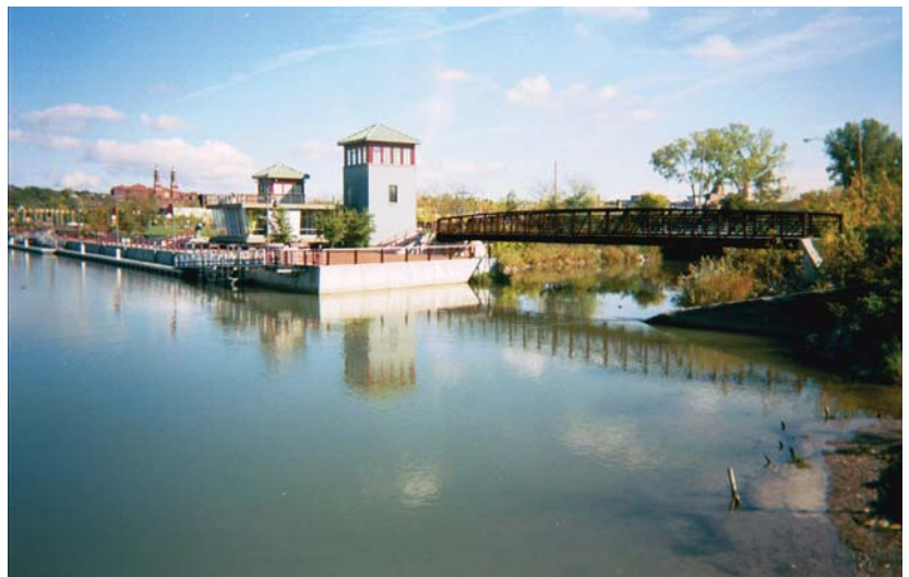
Photographs: Sections of existing creek walk, inner harbor, Syracuse
