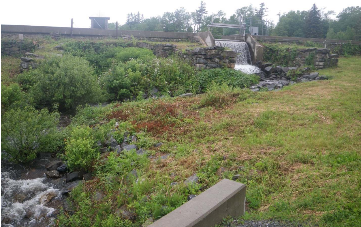
Figure 8. Water control structure at the outlet of Dyken Pond. (Photo credit: OEI)
