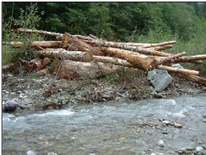
Figures 20 and 21 – In-bank Log Shelter ( http://www.mostateparks.com/jshutins/pics_riverrest.htm , Washington Department of Fish and Wildlife 2004)
